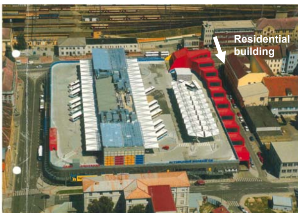
Fig.1. Aerial photograph of the investigated building and the coloured neighbouring obstacle
