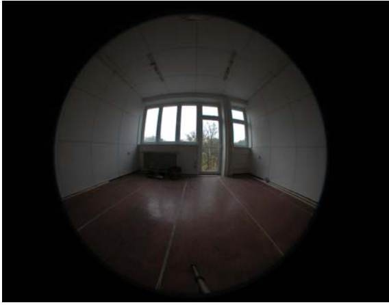
Fig.2 View on the window wall
